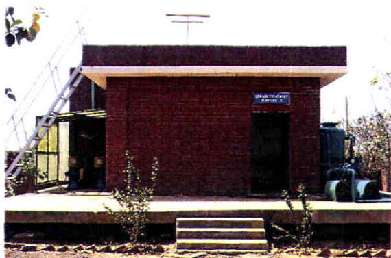
Sewage Treatment Plant (STP), at the campus
